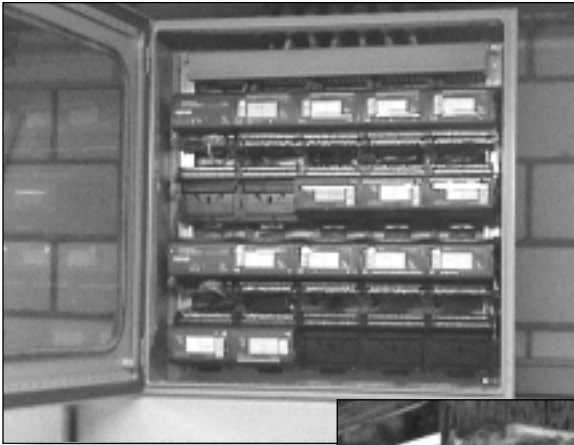
Left, two banks of FieldPoint I/O modules in a protected casing. Right, the crane operates day and night mixing the compost.
